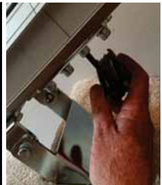
SLIDE BOTTOM JOINTING PLATE UP TO STRADDLE BOTH RAILS & TIGHTEN.
