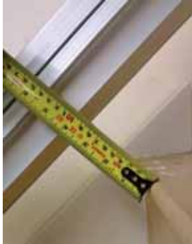
RAIL TO STEP NOSE MINIMUM OF 3 1/4"
