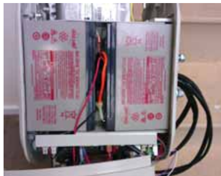
BATTERIES ROTATE BACK IN PLACE
