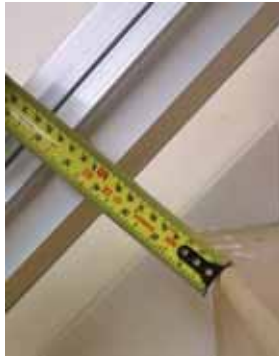
RAIL TO STEP NOSE MINIMUM OF 3 1/4"
